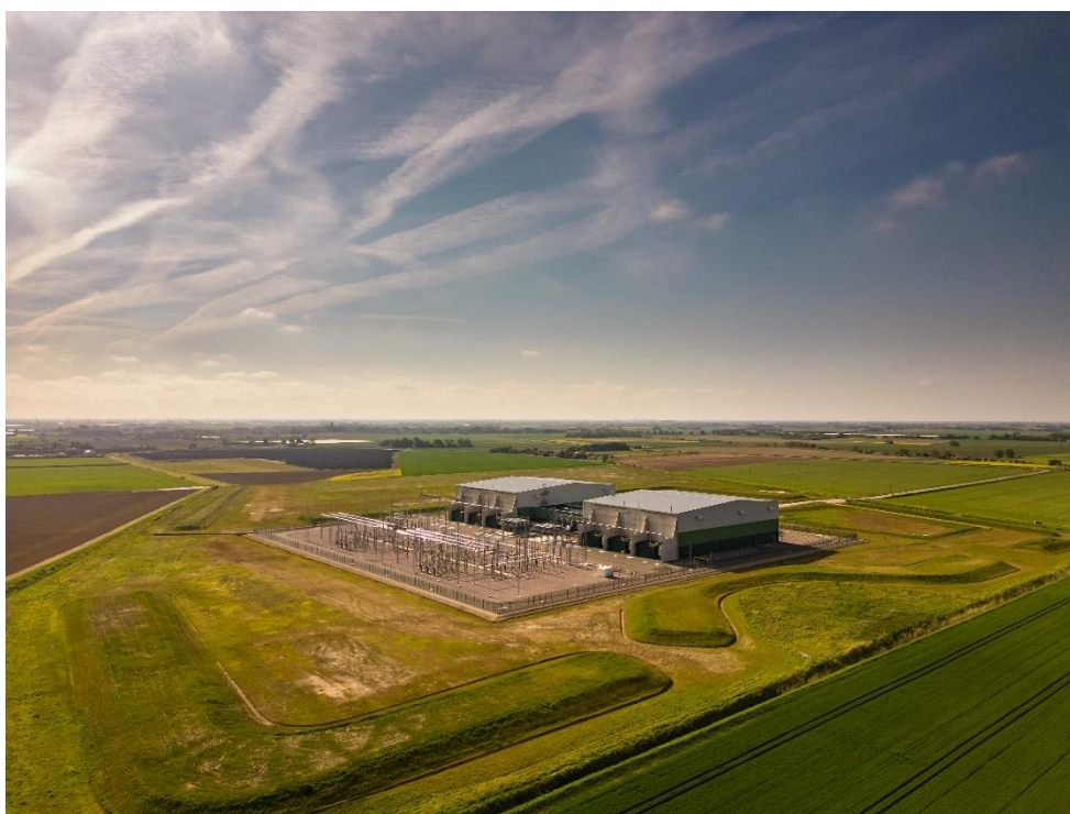
Figure 1.4: A 320 kV HVDC converter station. Source: National Grid
