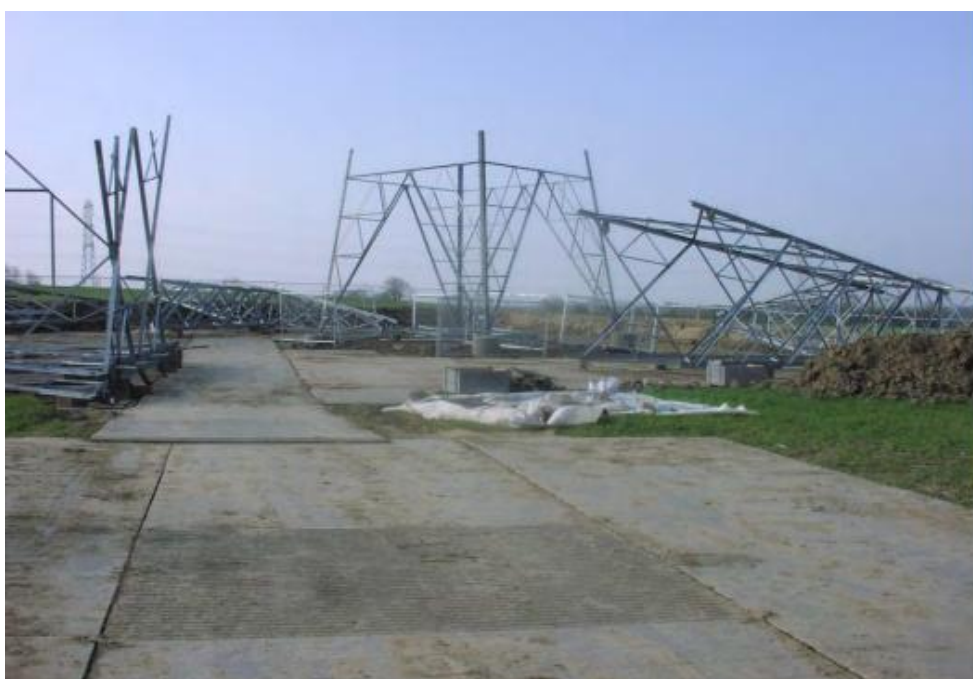
Figure 5.3: Pylon under construction. Source: National Grid
