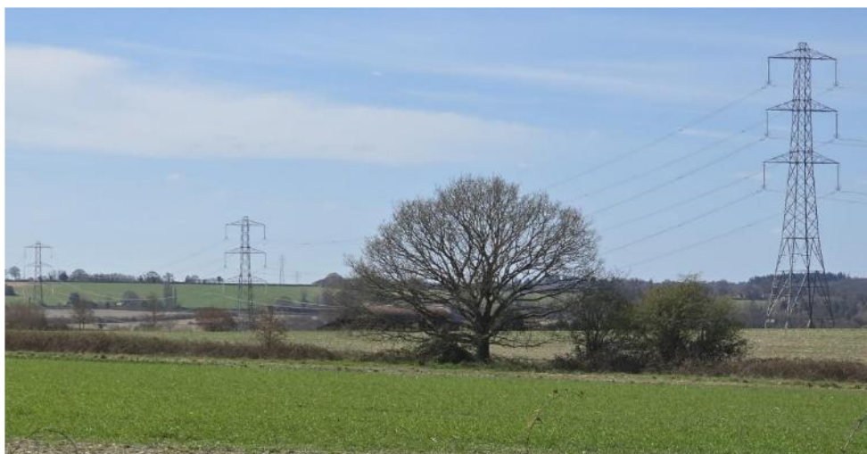
Figure 5.4: An OHL route taking lower ground to minimise ‘skylining’
