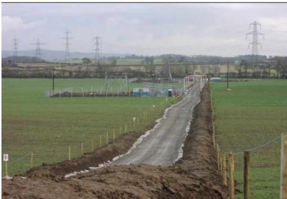
Figure 5.2: Temporary stone access track to pylon construction area. Source: National Grid
