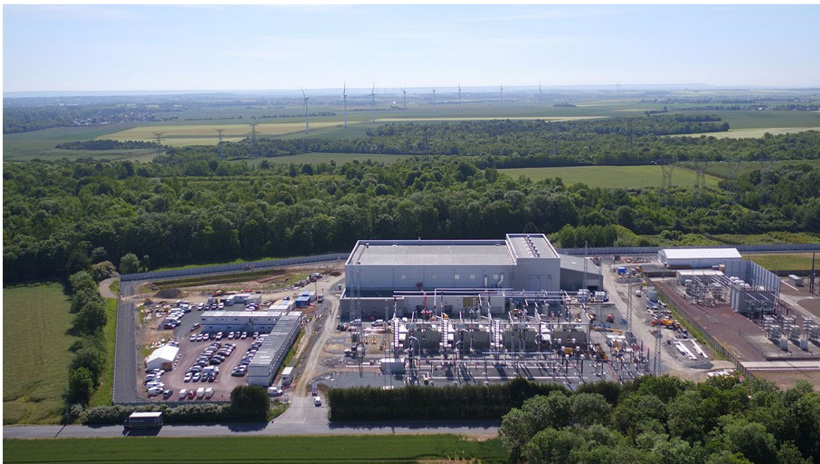
Figure 40: Example HVDC converter station
